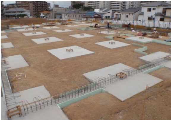
Fig. 12 Completed form of concrete foundation
