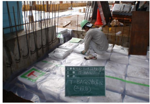
Fig. 14 Laying form of second layer under the floor
