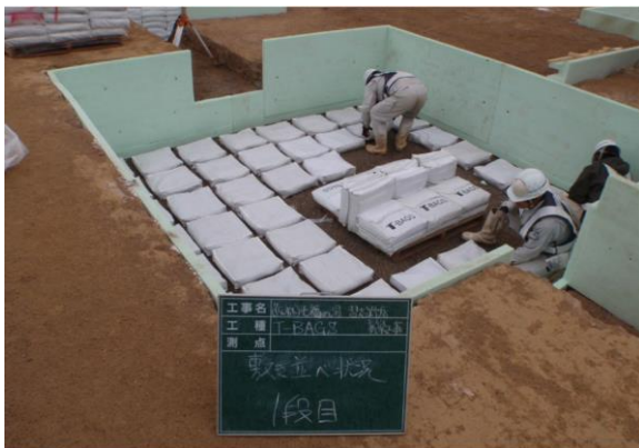
Fig. 7 First layer of T-BAGS are laying out
