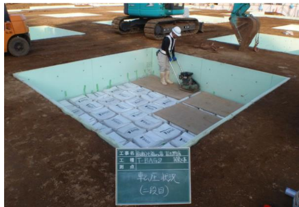
Fig. 10 Compaction situation of second layer
