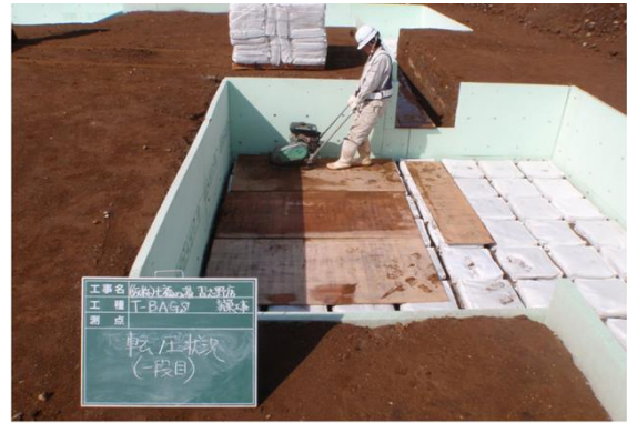
Fig. 8 Compaction situation of first layer
