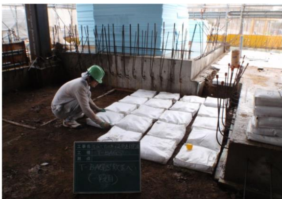
Fig. 13 Laying form of first layer of T-BAGS under the floor
