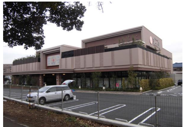
Fig. 15 Completed buildings construction
